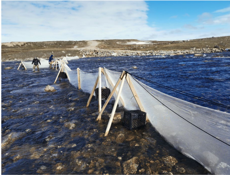
Figure 14. Clyde River restoration showing counting fence structure for video monitoring.
